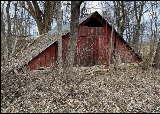
13. View of shed #2, northeast of the abandoned house, facing north.
