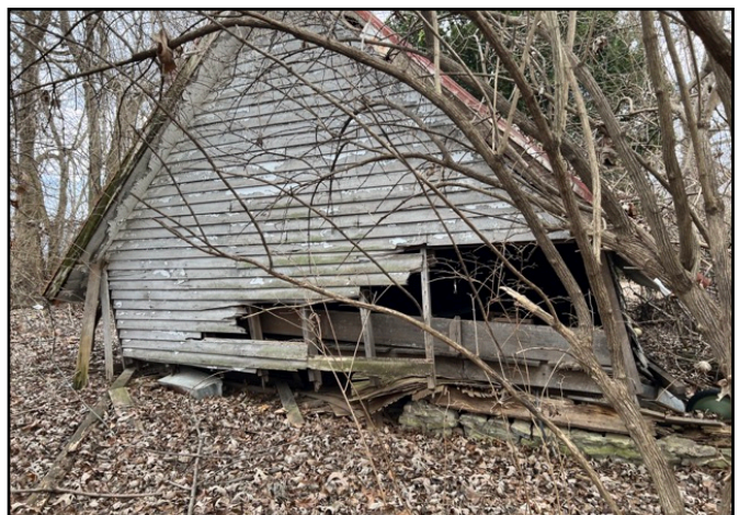
12. View of shed #1, west of abandoned house, facing west.
