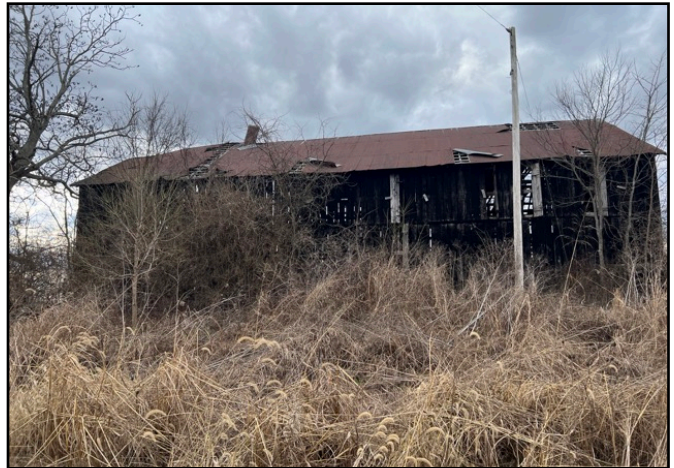
10. View of barn and power line. Facing west.
