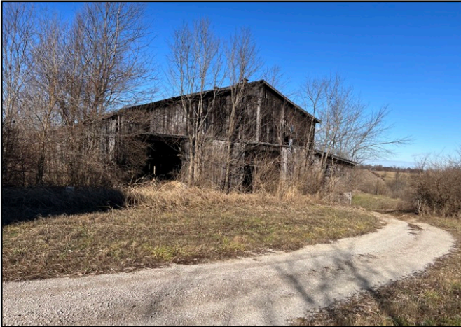
7. View of barn #1, in northwest corner, facing west.
