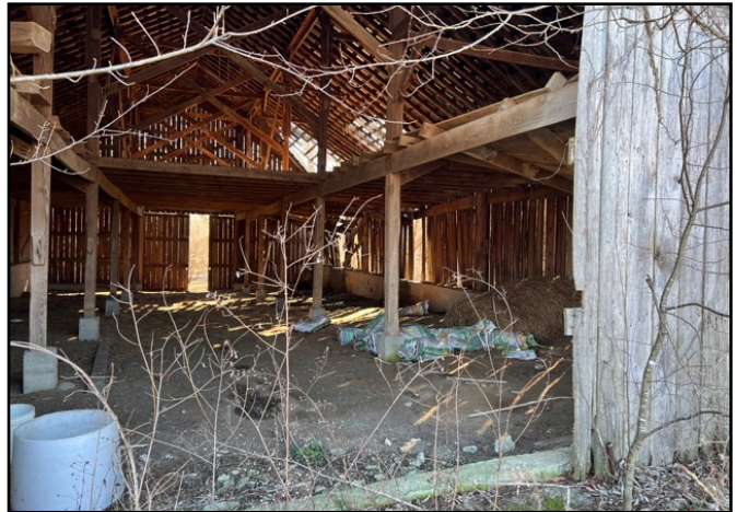
10. View of inside barn #2.
