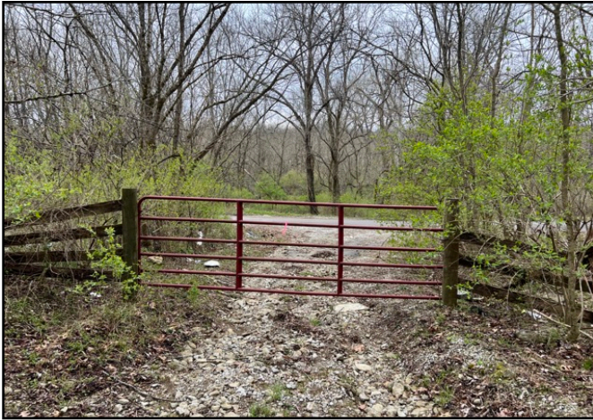
19. Example view of previous gravel road, with gate along Menelaus Road.
