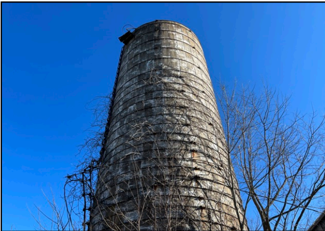
9. View of silo next to barn #2.
