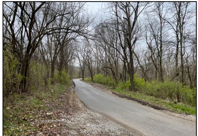
6. View of Menelaus Road, running along southern property boundary. Facing east.
