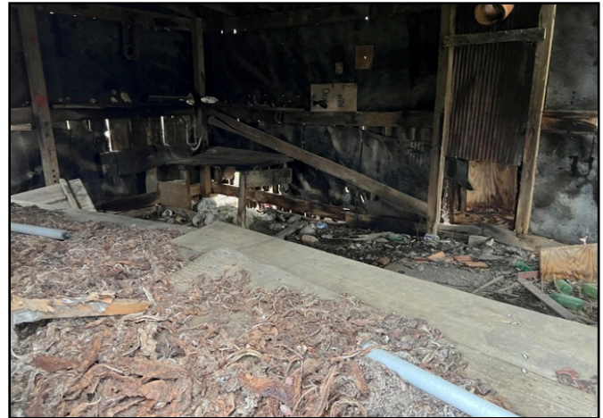
16. View inside shed #2.
