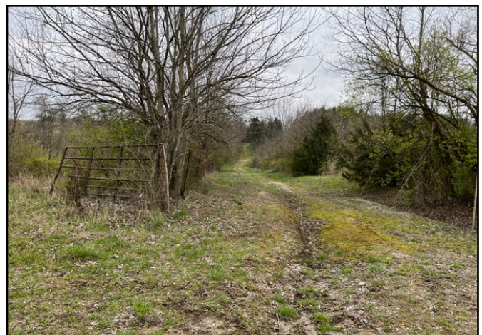
6. View of gravel road leading to neighboring property.
