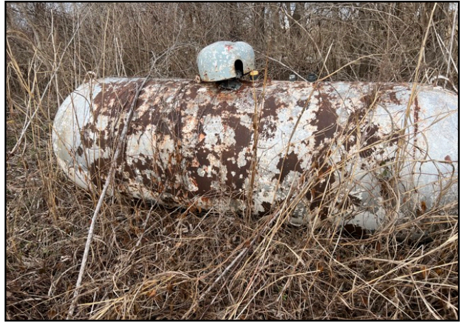
2. View of butane gas tank at northwestern section, facing north.
