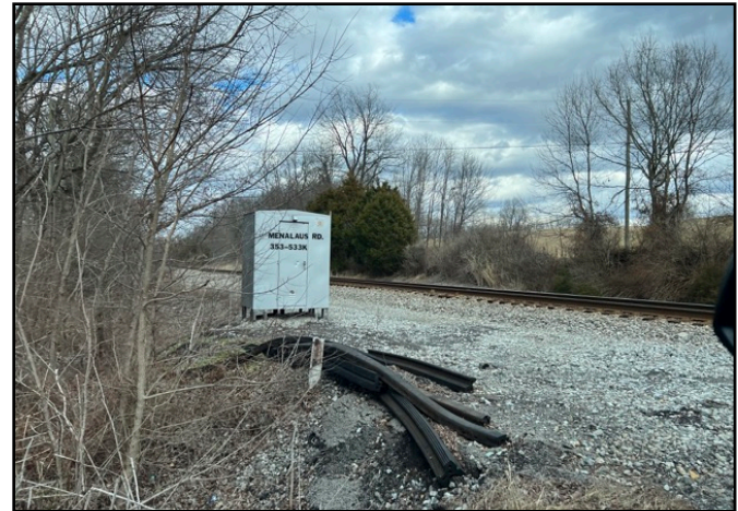
4. View of railroad tracks that run along western property boundary.
