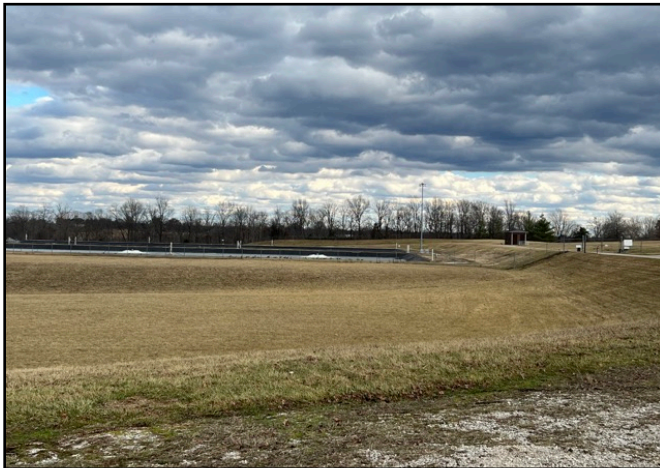
3. View of waste water treatment plant, south of the property.
