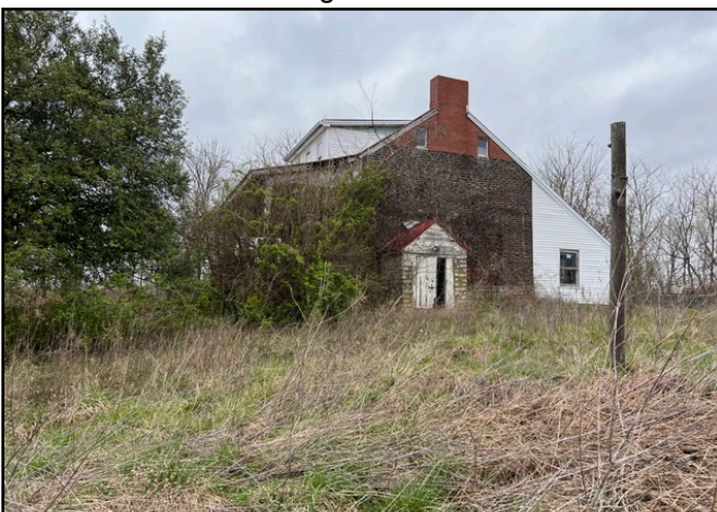
11. Example of abandoned house, facing west.
