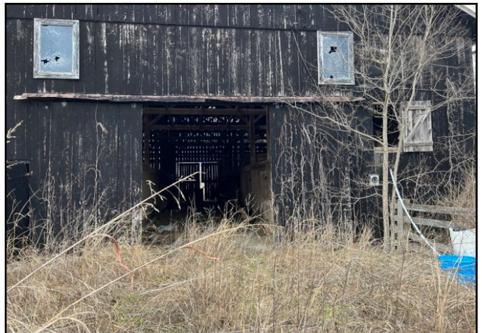
6. View of barn #3, which lies adjacent to barn 2, facing north.
