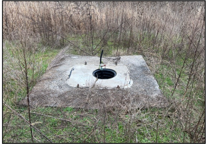
8. Example of small concrete pad with "manhole".
