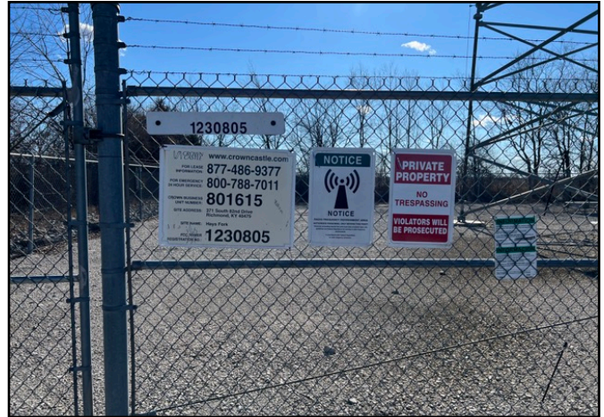
14. View of telecommunications tower showing fence and private property.
