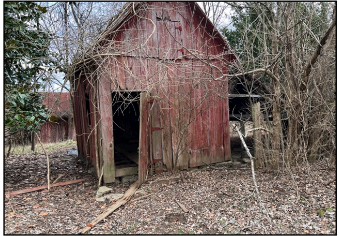
14. View of shed #3, east of the abandoned house. Facing east.
