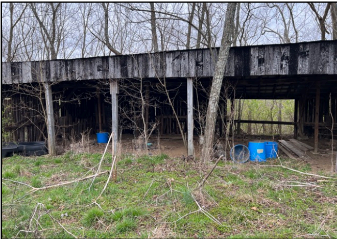
15. Example view of inside shed #1, facing southwest.
