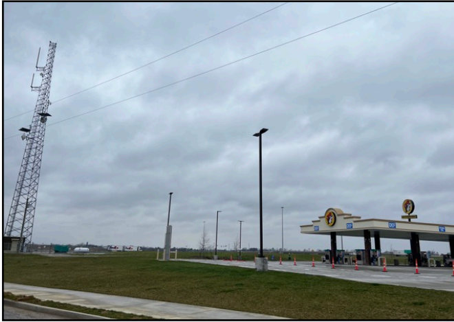
1. View of Buc-ee's gas station northeast of the site. Also showing communications tower, and above ground storage tank next to the tower. Facing northeast
