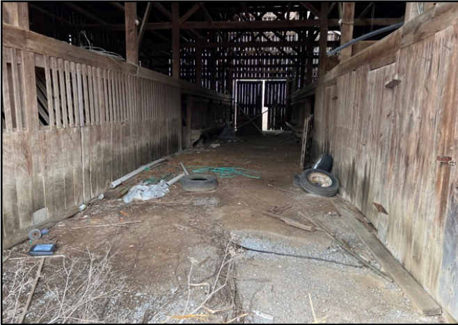
7. View of inside barn #3.
